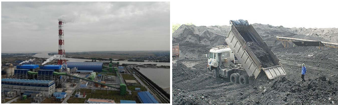
Figure 1. Thermal power plant and ash slag emissions
