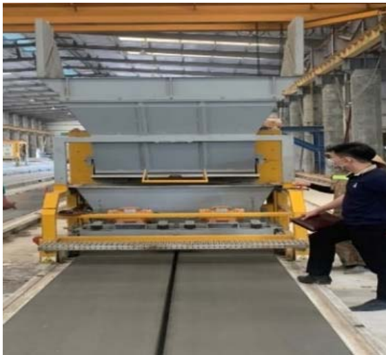
Figure 4. Fabrication of precast concrete hollow wall panels using extrusion technology
