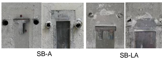
Figure 7. Shear bracket and beam socket after tested
